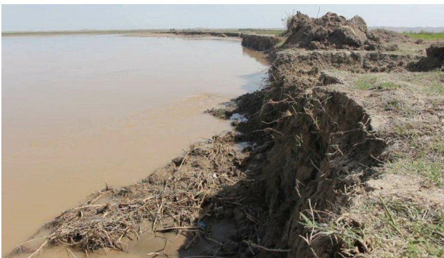
Figure 2-1 Amu River Bank Erosion [5]
